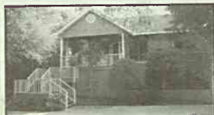
Coral Ridge Road, Beacon's Reach
