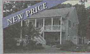
288 RAMSEY DRIVE NEWER CUSTOM BUILT HOME 9 FT CEILINGS THROUGHOUT
