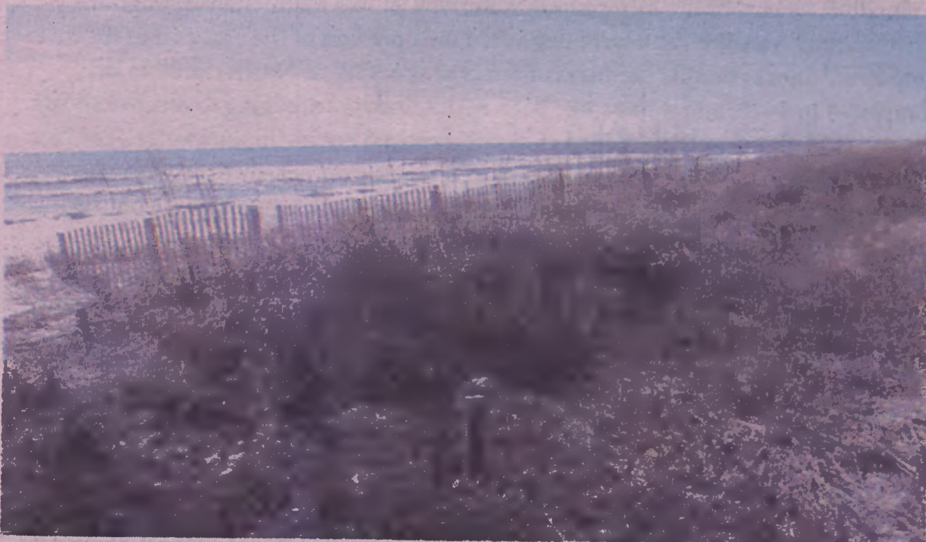
Top, work performed during the 2013 beach renourishment project in Pine Knoll Shores and, below, good results achieved from sand fencing and planting of beach grass.—Photos by Brian Kramer and Walt Zaenker
