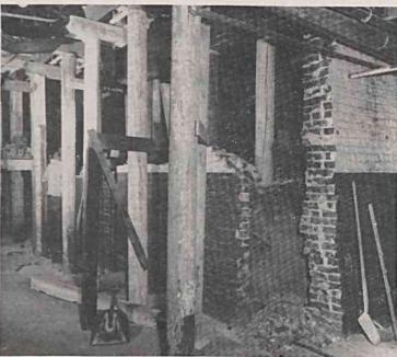
Brick wall shown at right has now been removed. Steel columns are to support roof and roof beams. New scouring machine will extend toward left in picture virtually all the way across the former boiler room space. Outside doors to boiler room have been bricked up. Building alterations amount to a major remodeling job.
