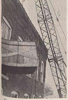
C. E. Martin (Engineering), whose hobby is photography, snapped this picture as a 20-ton portable crane lifted a crated IBM machine to the Tabulating Dept. on the second floor of the General Office. Two machines formerly in use were removed and replaced by hew, more modern equipment.
