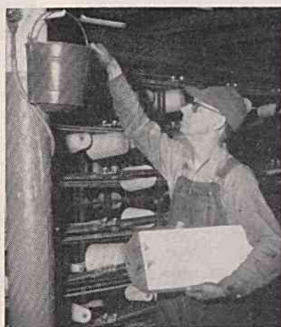
I. H. Shively, of Karastan shop, has inspected all valves and now checks fire buckets to make sure water is available for extinguishing small fires.
