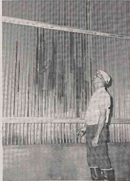
Homer C. Vernon, humidifier and cleaner repair man at Bedsread Mill, observes stainless steel eliminator blades used with evaporative cooling system.
