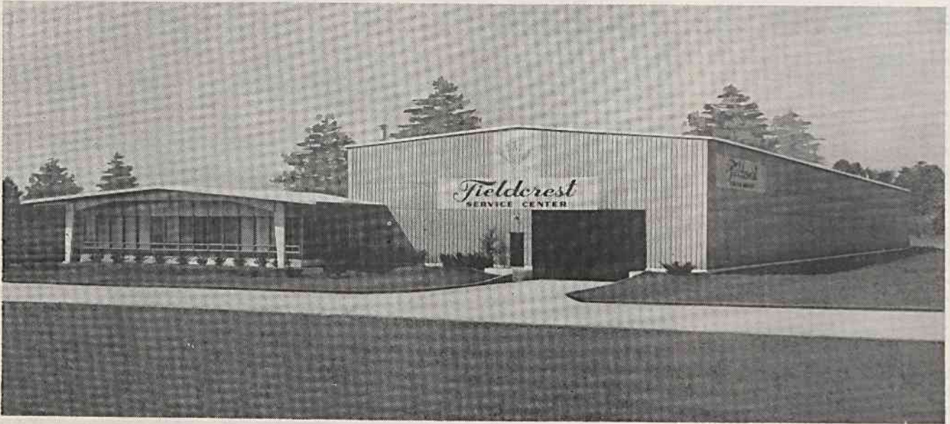
This large and modern building in suburban Cleveland houses Fieldcrest's newest and largest customer Service Center.
