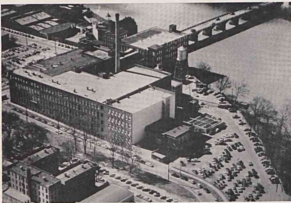
Muscogee Mills, a Unit of Fieldcrest Mills, Inc. has all operations in one plant location. This view shows the mill buildings on Chattahoochee River in Columbus.
