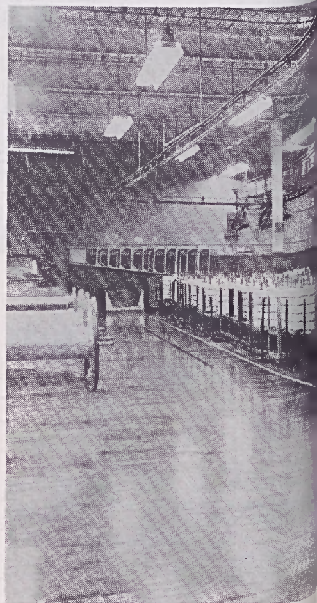
Excellent zoning in Spooler Room provides for efficient operation and other movable equipment are stored in an orderly manner.
