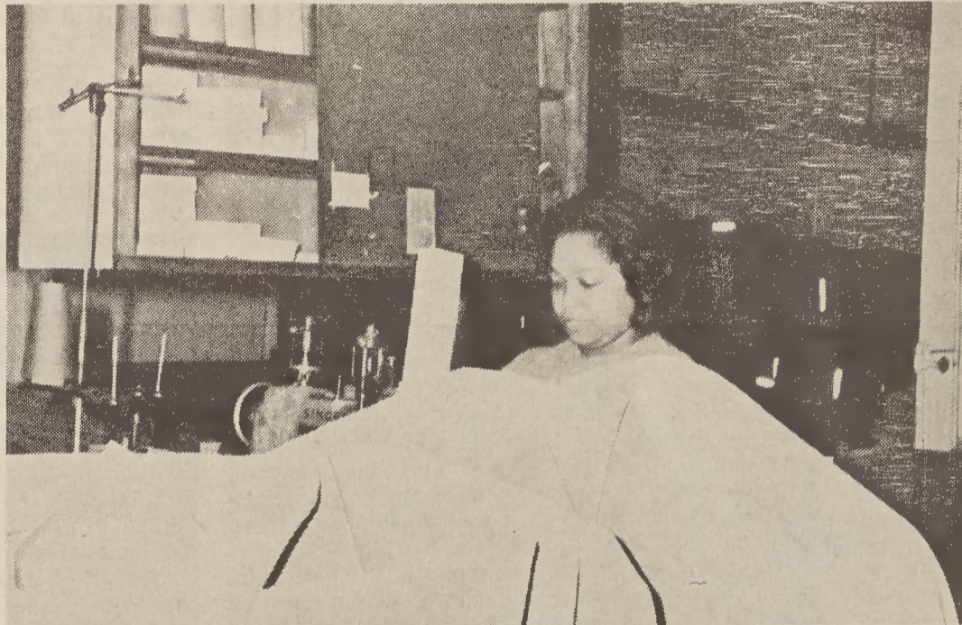
GLADYS KING — Sewer-Blankets, Cut and Sew Department
