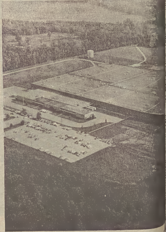
The Bedsread Finishing Mill, right, adjoins the Sheet
