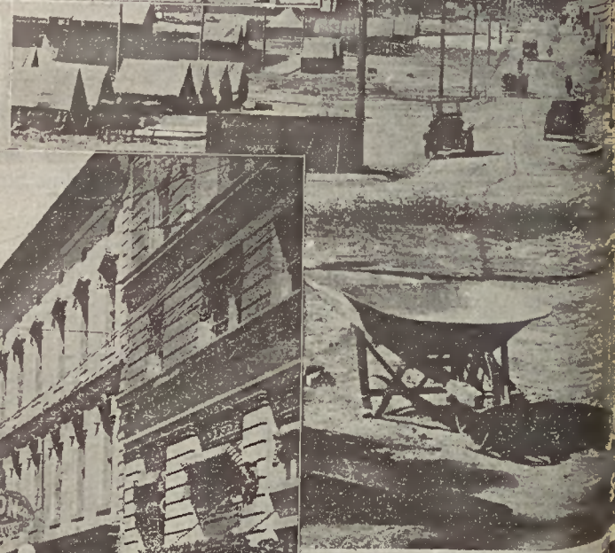
Construction going on
