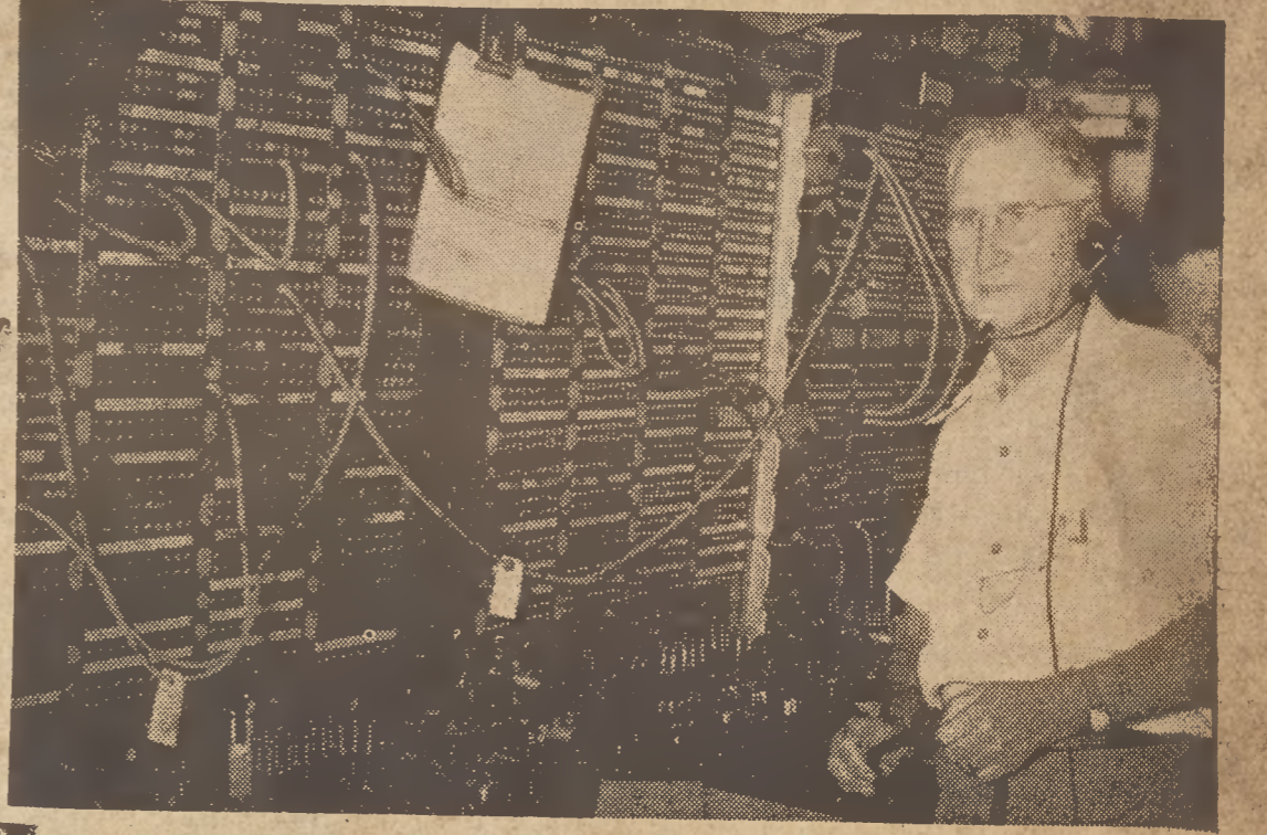
J. C. Diehl, test board man is shown at the large test board in the Selma station. On this board wire trouble is located between Selma and Richmond and Selma and Denmark, S. C.
