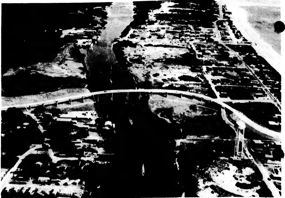
Above is an aerial photo with an artistic rendering of the future bridge over the intercoastal waterway at Holden Beach designed by Bigger and Agnew, Inc. engineers of Raleigh.
