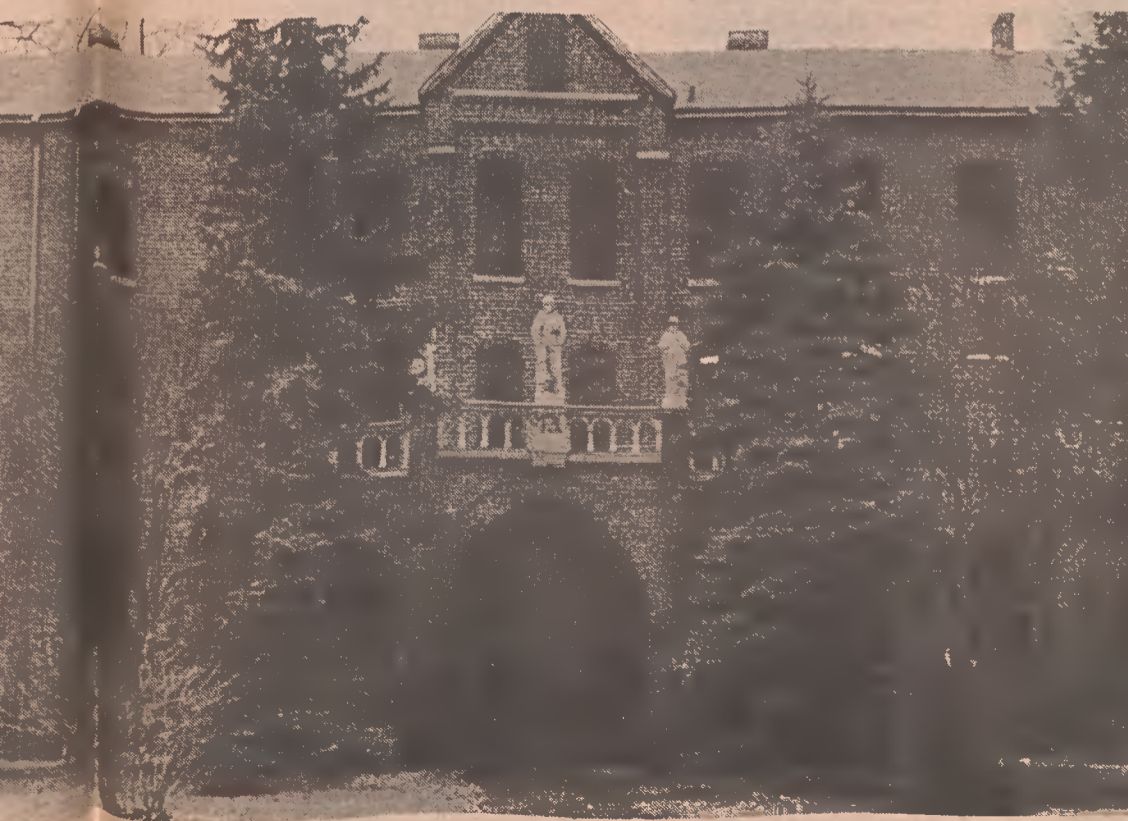
AFTER RENOVATION, here is the entrance at the front of the building.
