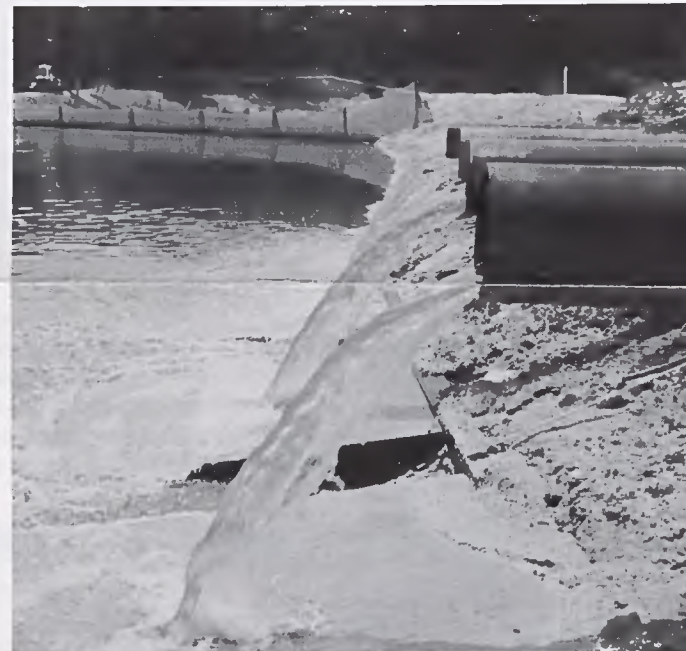
Clarified water is pumped back into settling pond.
