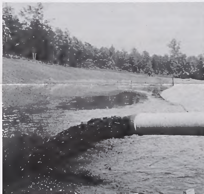
Black sediment is pumped into receptor basin
