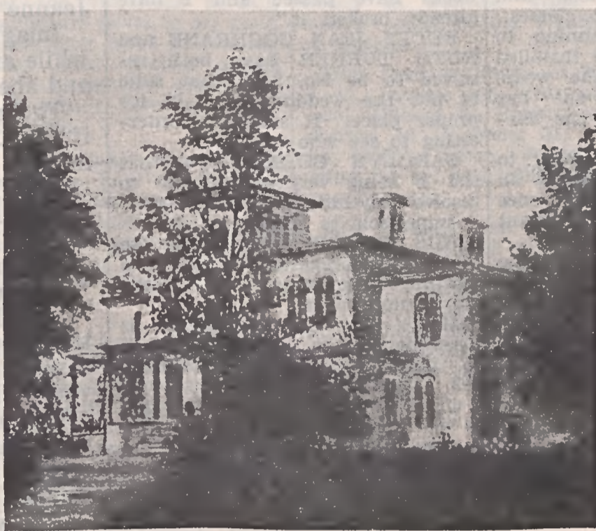
QUEENS ON COLLEGE STREET
