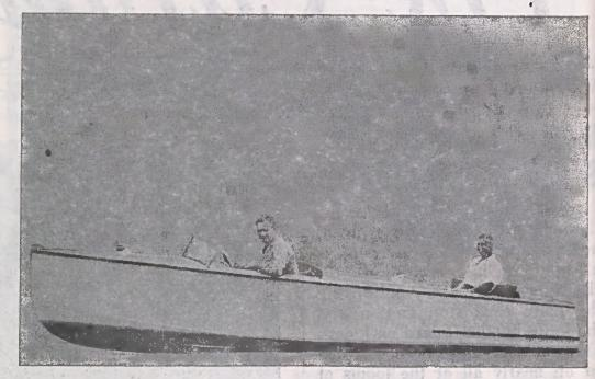
Shown above are Ledford Waters and Leslie Alexander of the Weavershed in a motor boat that they had just recently completed costing approximately \$1,800.00. They started the boat in January; and built it in Leslie's backyard. Practically the only tools that were used were a hammer, chisel, screw driver, and a drill.
