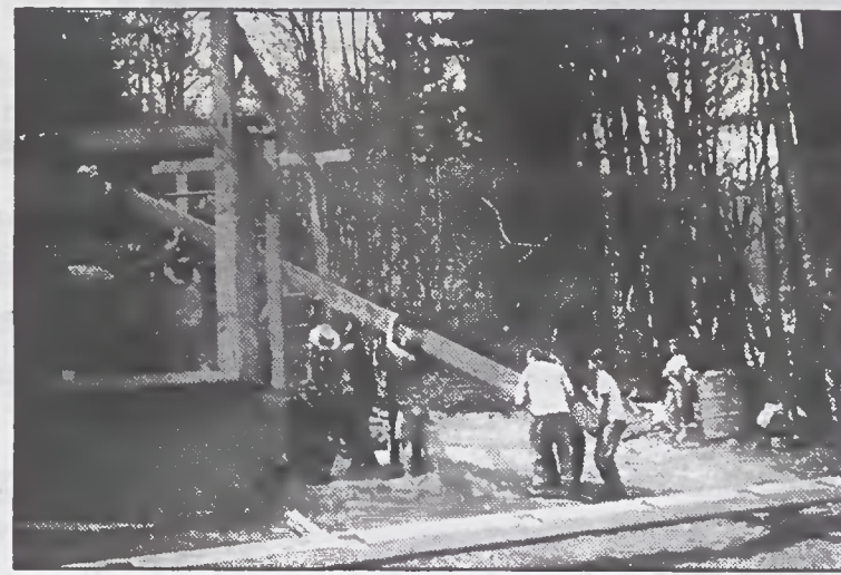
Workshop students raising the frame for the ICE House in 1989.
