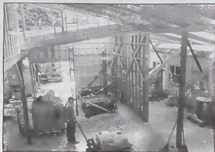
Inside the new kiln shed.
