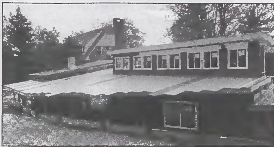
The almost complete kiln shed.
