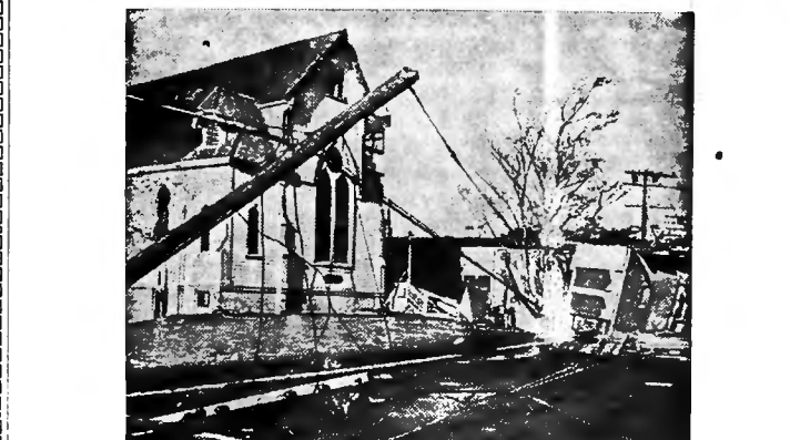
The big blow twisted the steeple off this Massachusetts church and toppled it into the street across the electric wires. Another headache for hard-working linemen!
