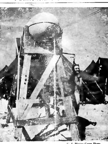
Marine ingeniously took a badly-damaged belly gasoline tank and patched it, then placed it atop some Japanese lumber and thus provided a shower bath on one of the Pacific Islands group.
