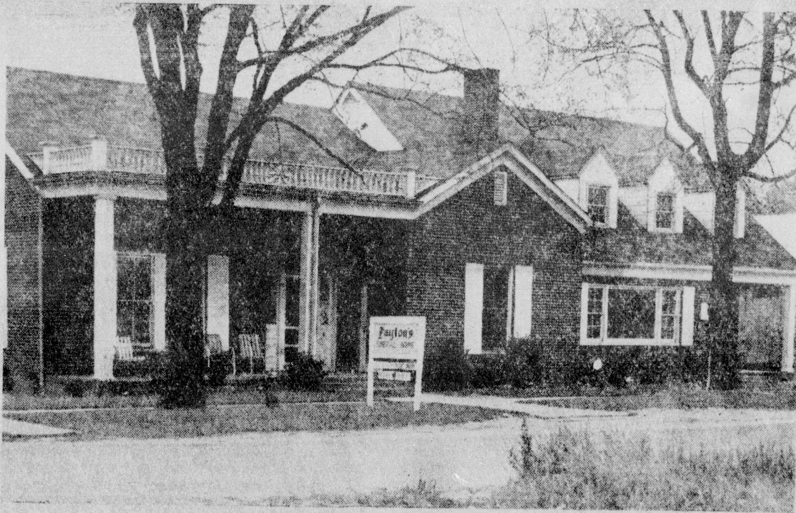
DEDICATION HELD — Above is shown the newly completed O. S. Payton Funeral Home at 101 East Harnett Street in Dunn, N. C. More than 500 persons from Harnett, Sampson, Johnston and Cumberland Counties were present Sunday afternoon for open house and dedicatory exercises for the 21-room building which features a spacious chapel and complete facilities for the most careful and dignified of funeral services.
