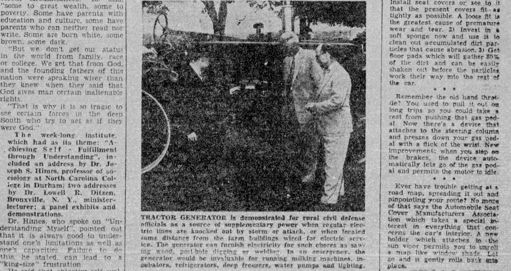
TRACTOR GENERATOR is demonstrated for rural civil defense officials as a source of supplementary power when regular electric lines are knocked out by storm or attack, or when located some distance from the farm buildings wired for electric service. The generator can furnish electricity for such chores as sawing wood, post-hole digging or welding. In an emergency, the generator would be invaluable for running milking machines, incubators, refrigerators, deep freezers, water pumps and lighting.
