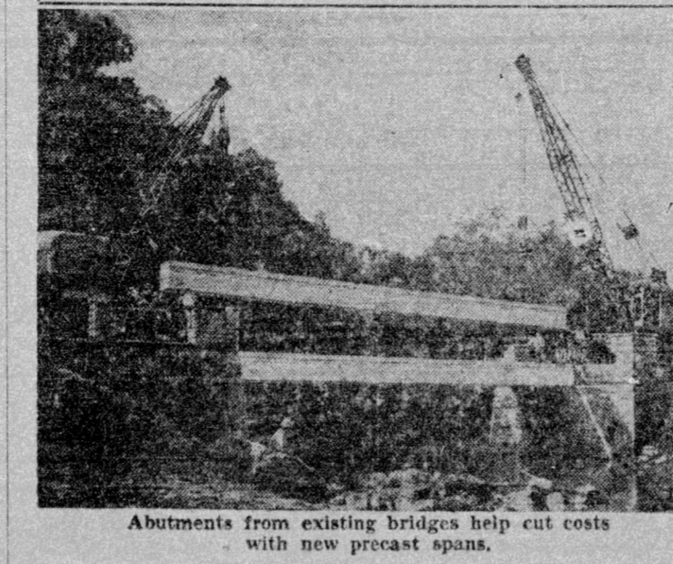
Abutments from existing bridges help cut costs with new precast spans.
