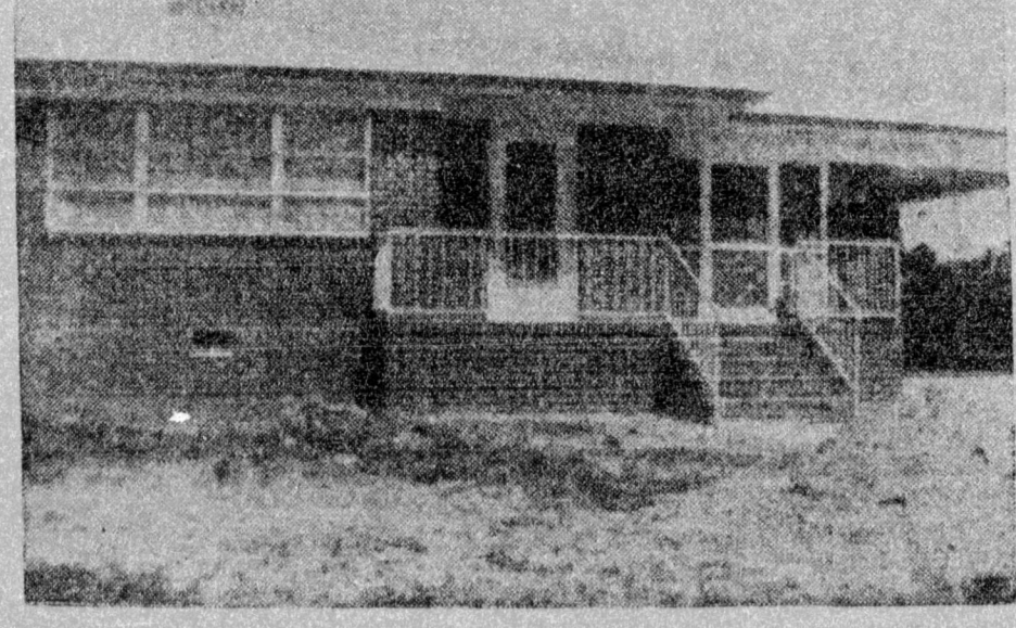
THE NEWLY BUILT ROBINSON HOME
