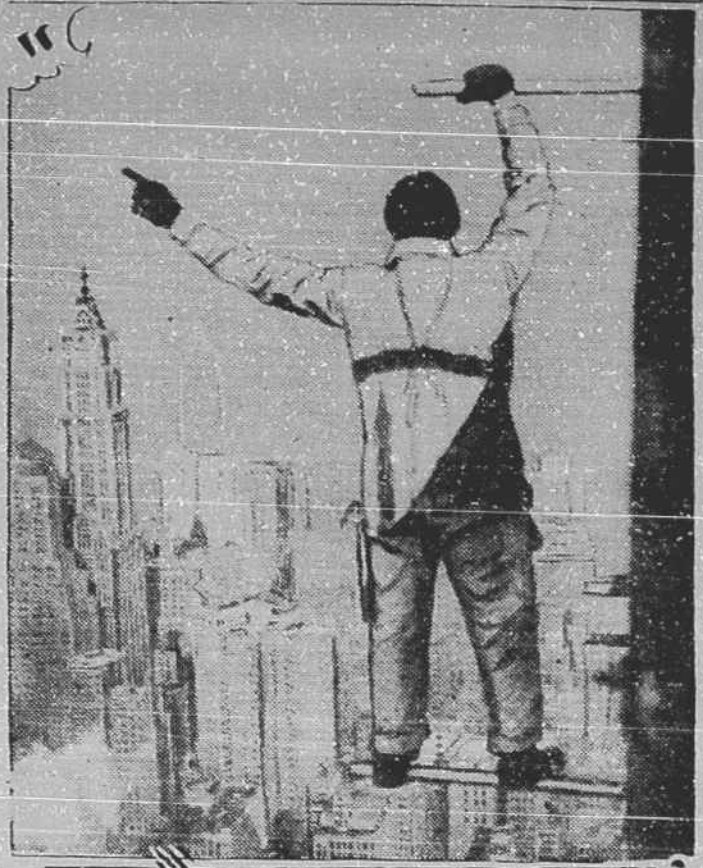
M. P. Doherty, a Brooklyn steel erector, swinging out from the 69th story of the new Bank of Manhattan building in Wall Street, to look down on the Woolworth Tower and the money center of the world. The New York Stock Exchange is the low building in the center of the picture.
