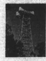
side or on a hill, with the horn-like contraptions on top. Well, radio relay bounces your voice across the country with the speed of light from tower to tower, spaced about 30 miles apart. It supplements land wires and carries hundreds of telephone conversations at the same time. Radio relay is still another way we're working together to bring people closer together.
