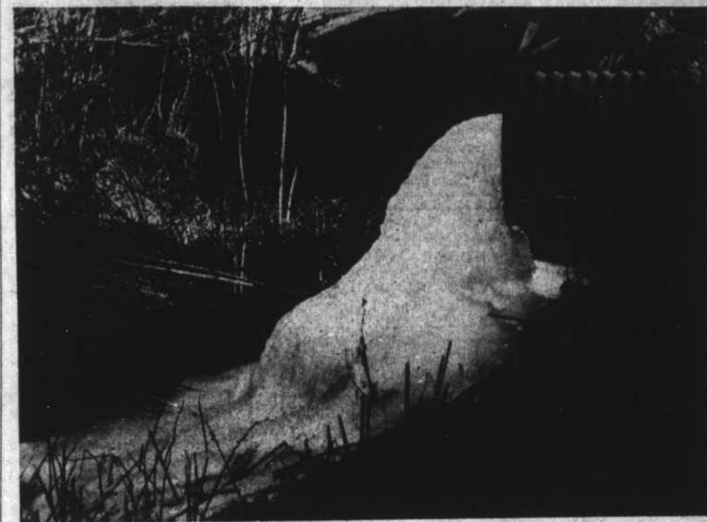
WAS IT THAT COLD?—Highway engineers estimated that nearly a thousand pounds of ice projected from this culvert under U. S. Highway 321 near Boone at the time this picture was taken. Resembling a huge ice machine, the water froze as it drained into the creek below the road.—Photo Flowers' Photo Shop.
