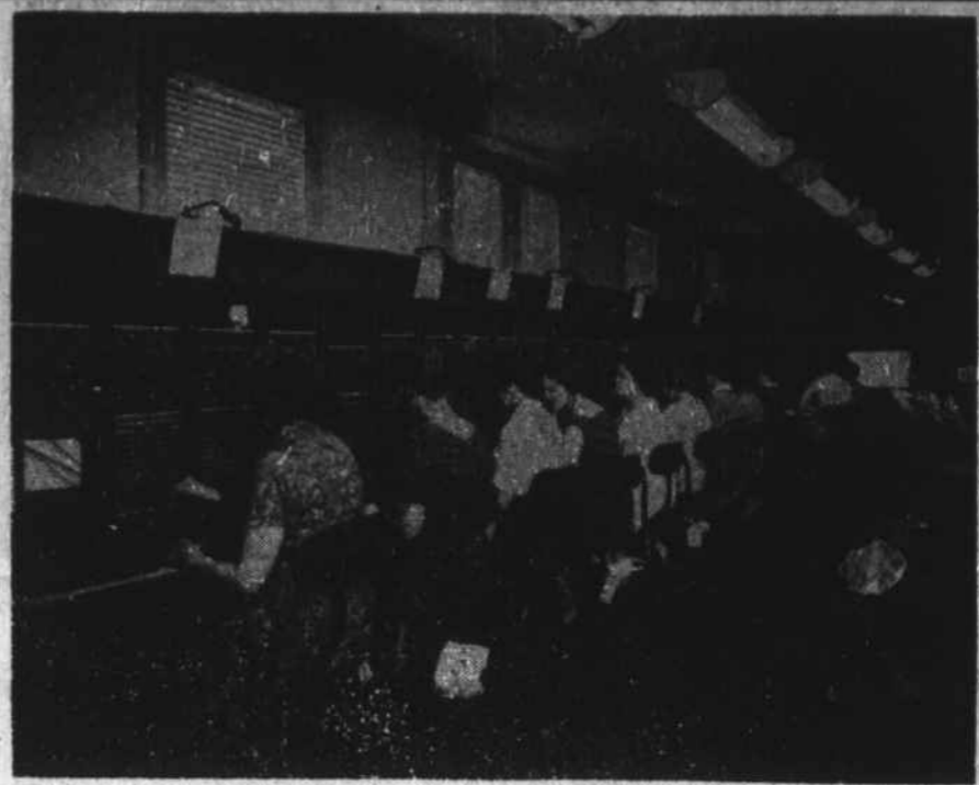
THE END OF AN ERA—On early Sunday morning, June 25, this manually operated switchboard closed and local calls for Hamlet were handled by modern electronic switching equipment. When Hamlet cut over to dial service Southern Bell was 100 per cent dial in the exchanges it operates in North Carolina.
