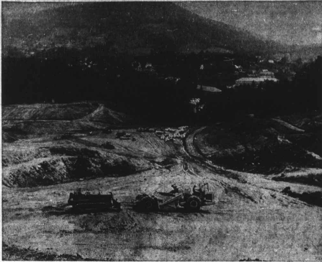
GRADING FOR APPALACHIAN STATE TEACHERS COLLEGE STADIUM IN PROGRESS.
