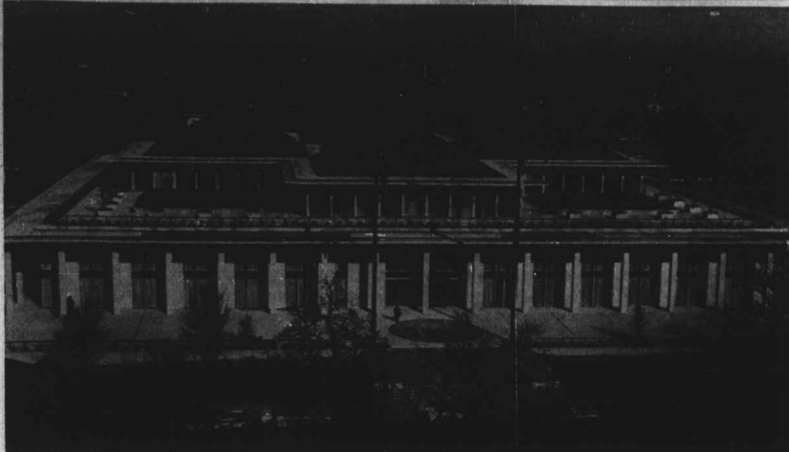
NORTH CAROLINA STATE HOUSE.—The new State House in Raleigh will be open to visitors after the 1963 General Assembly convenes on February 6. The first building ever constructed by any state for exclusive use of its Legislature was designed by Edward Durrell Stone of New York.—State News Bureau photo.
