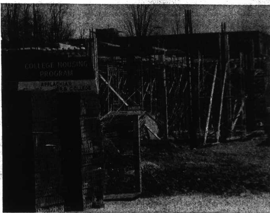
ASTC STUDENT CENTER—Despite a recent illness of George Durden, Superintendent for Juno Construction Company, and the fact that several workers have been out with influenza, the foundations are in, and
