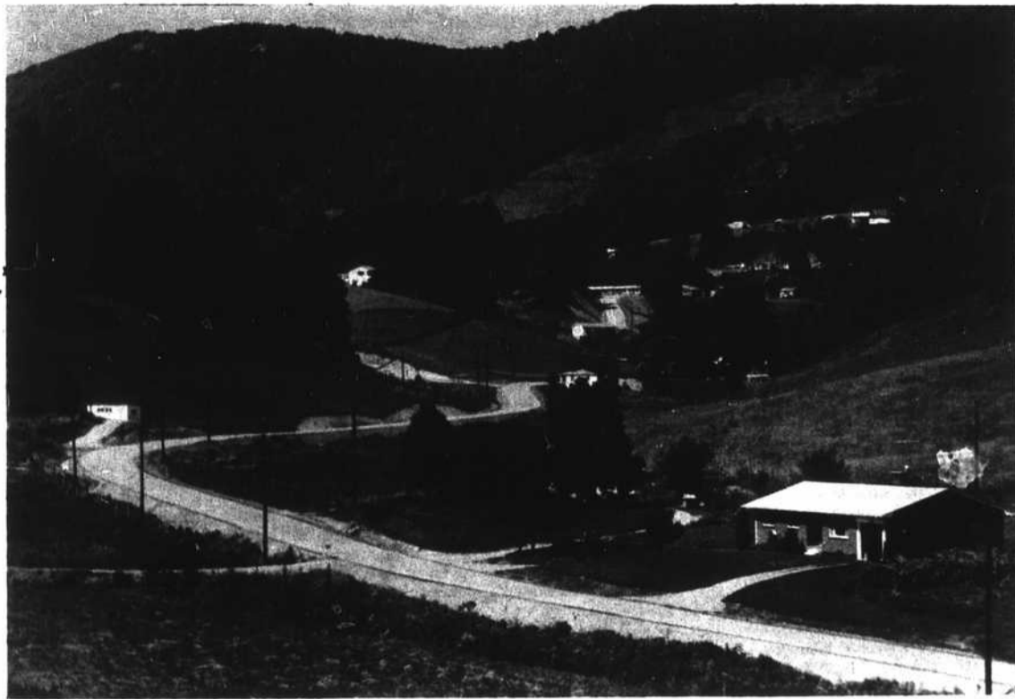
THE GEORGE WILSON ROAD is nearing completion. It is one of four secondary roads in Watauga County which presently are being hardtopped at a cost of $59,792. Highway Engineer Tom Winkler says the grading on the roads was done by the State Highway Commission and contractor for the paving is a Mt. Airy
