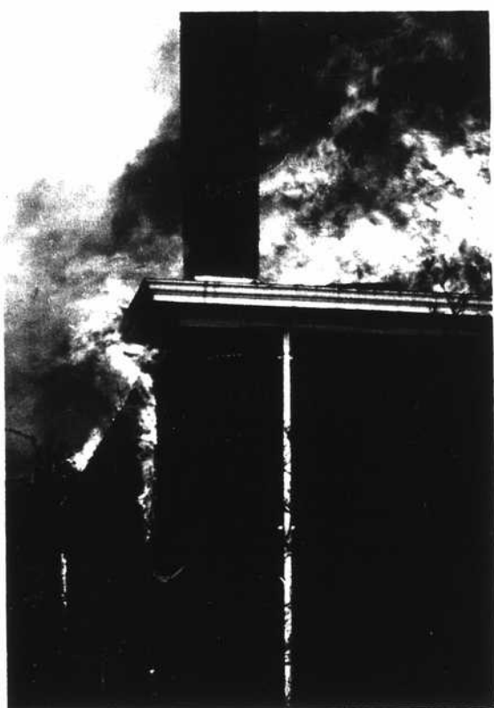
Flames burst from the roof of the administration building on the Appalachian State Teachers College campus.
