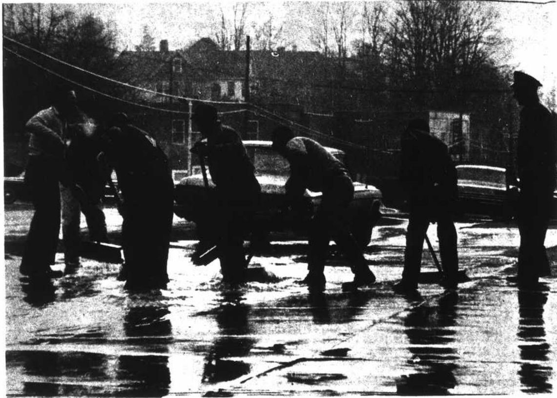
Hydrant's On And Work Begins
