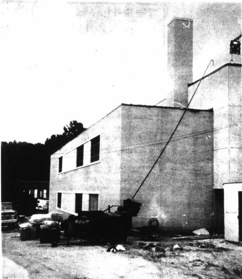
NEAR COMPLETION —Watauga's new courthouse on West King Street is in the final phase of construction and expected to be occupied sometime in October. Claude Danner, Tax Supervisor and clerk to the Board of County Commissioners, says the architect and contractor reported the progress to the Board Monday but set no definite date when a move could be made from the temporary courthouse in Junaluska Heights. In the court room, the paneling nearly is completed; the jury box, witness stand and judge's bench are in place; and the divider between the bar and the spectators is finished. Hallways and offices on both floors are reported finished, but the tile floor in the court room is not yet laid. Upstairs wash rooms are tiled and most of the work done downstairs where also, the ceilings are being lathed for plaster. A lot of electrical work remains to be done, according to Danner. This scene is from the back of the building looking toward main street. Temporary closure of the roof has been done and permanent sealing is to be accomplished this week. (Staff photo)
