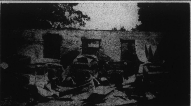
AFTER THE FIRE—This is an inside scene of the Charles H. Jenkins and Co. building in Aulander after it was destroyed by fire in 1923.
