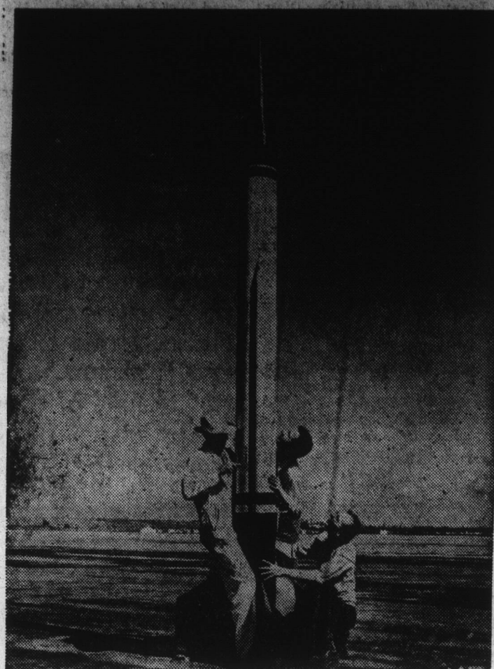
ALL-AMERICAN ROCKET—THE WAC CORPORAL—is smaller than the 14-15 ton German V-2. Developed in 1945, the experimental, liquid-fuel, high altitude rocket weighs 655 pounds with a full fuel load and attains a top speed of approximately 2,800 miles an hour.
