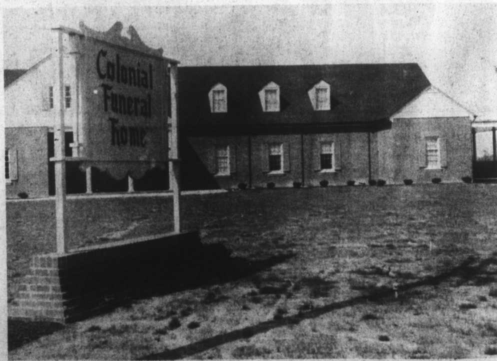
NEW FUNERAL HOME —Formal opening of Colonial Funeral Home on Highway 32 North will be held Saturday and Sunday from 2 P. M. to 5 P. M. The new funeral home is described as one of the most modern in Eastern North Carolina. Built by Edenton Construction Company, the new establishment will be managed by Marvin Barham, one of two licensed funeral directors and embalmers on the staff.
