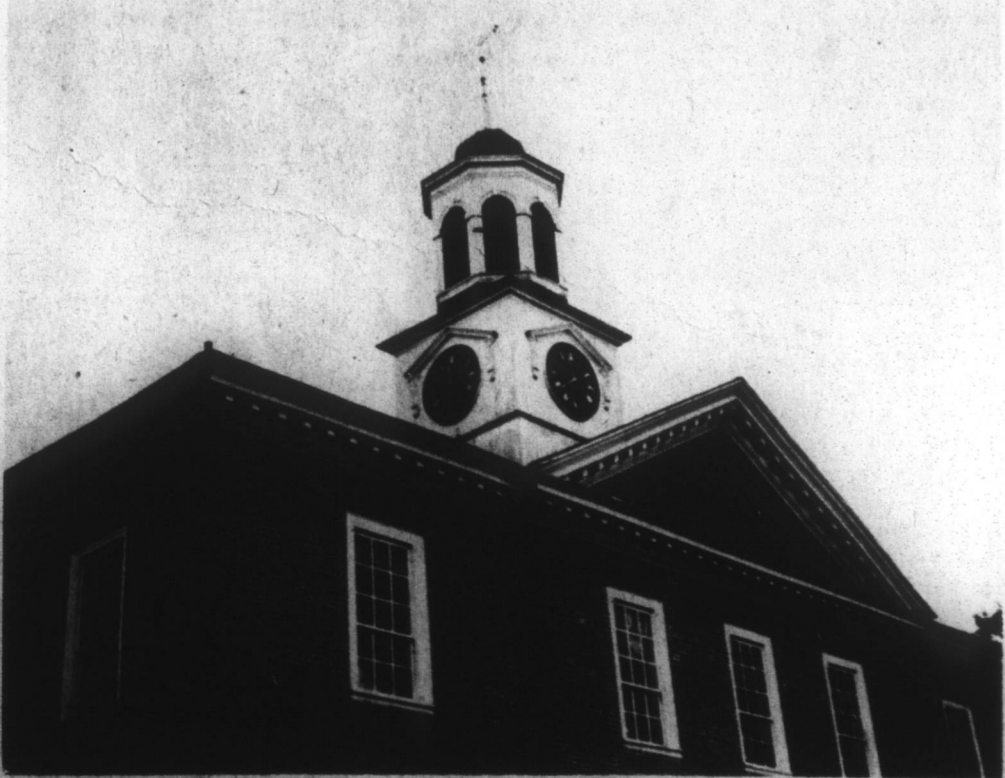
BACK IN SERVICE—Edenton again has an official time piece. The handsome old clock atop Chowan County's historic Court House was restored to service Monday, including the striking mechanism. Chairman W. E. Bond of county commissioners said the clock will strike every hour from 7 A. M. until 9 P. M. The striking was stopped several years ago and the entire clock went out of service during the winter's ice storm. A representative of Bedgood's Clock Service of Macon, Ga., repaired the time piece and reports it is one of the finest clocks in service today.
