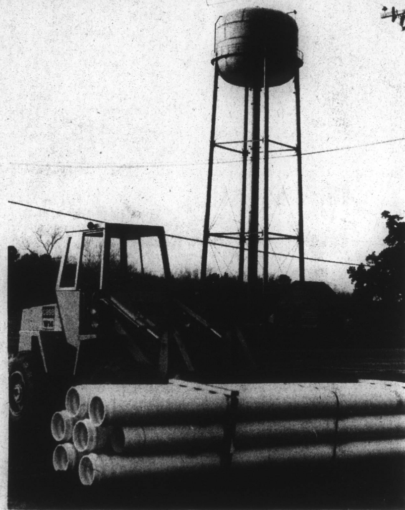
FIRST TANK ERECTED—The first tank in the Chowan County water system has been erected near Welch, on Highway 32 north of Edenton. It now stands ready for inspection and painting. Work on installing the pipe is nearing completion. (Allan Asbell Photo).
