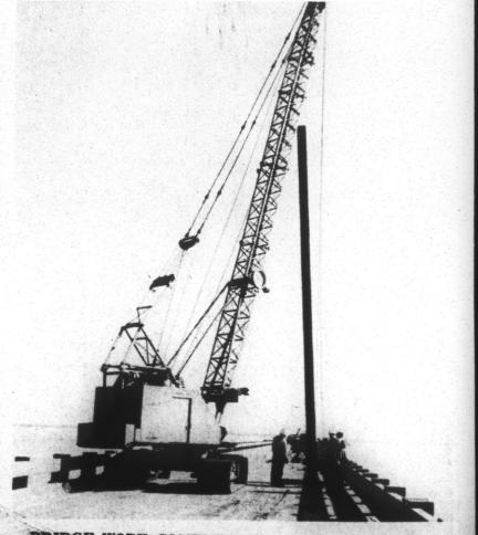
BRIDGE WORK COMPLETED - A huge crane aided the Department of Transportation bridge maintenance workers to install a new piling on Albemarle Sound bridge, east of Edenton. Ice in the sound severed or severely damaged dozens of wooden pilings, causing DOT officials to close the bridge to traffic in late January.
