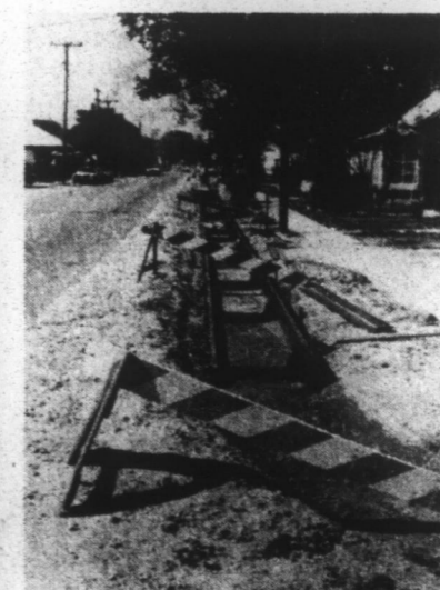
Curb And Gutter
