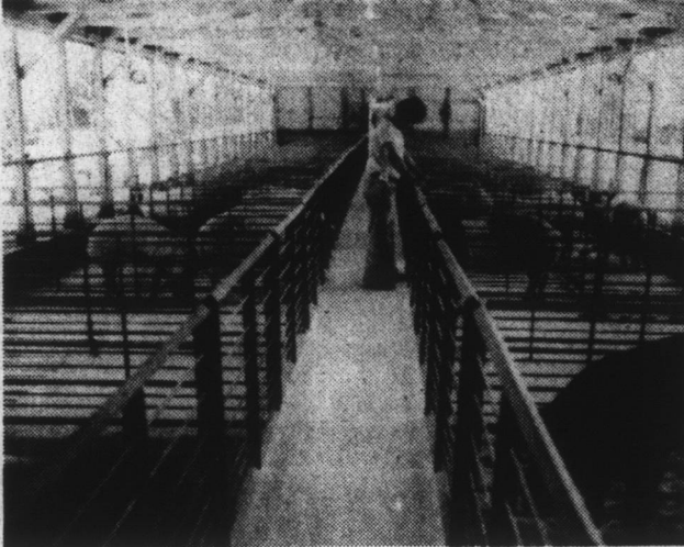
CONFINEMENT HOUSE - Neal Griffin, a new hog producer in Chowan County, looks over his first selection of gilts and boars. This is his sow confinement house with the farrowing house under construction. (SCS Photos.)
