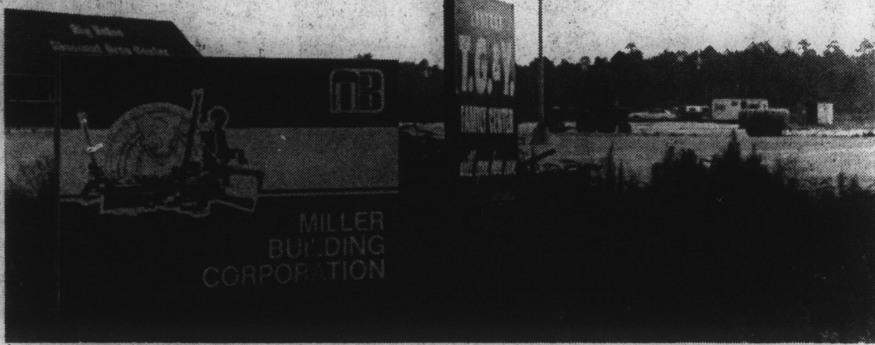
ACTIVITY AT SHOPPING CENTER —Work is now underway on a 77-square-foot addition to Edenton Village Shopping Center on North Broad Street. Also, new tenants are being signed for the first two units at the center, now owned by Figure Eight Development Corp., of Wilmington. (Staff Photo by Luke Amburn.)
