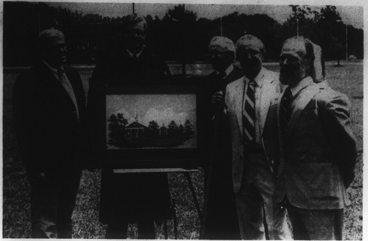
SANCTUARY PROJECT UNDERWAY — Groundbreaking ceremonies were held Sunday morning for the sanctuary addition to Edenton United Methodist Church on Virginia Road. It is expected to take 13 months to complete the $800,000 project. Pictured left to right at the ceremony are: L.F. Amburn, Jr., Building Committee chairman; Rev. Kermit Braswell of Elizabeth City, district superintendent; Rev. Richard Blankenhorn, pastor; Will Parker, trustee chairman; and D. Ross Inglis, president, Edenton Construction Company, Inc., general contractor. The Fellowship-Education Building was started in July 23, 1978, and occupied in mid-1979. When the sanctuary is finished the church will have a $1,250,000 investment adjacent to Chowan Hospital. (Staff Photo by Paul Amburn.)
