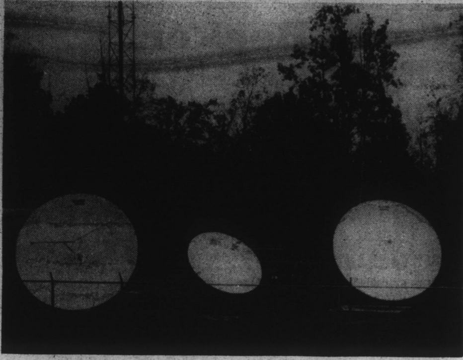
NEW DISH—Pictured here are all three of the dishes installed by Albemarle Cable TV to bring its customers a total of 27 channels from which to choose.
