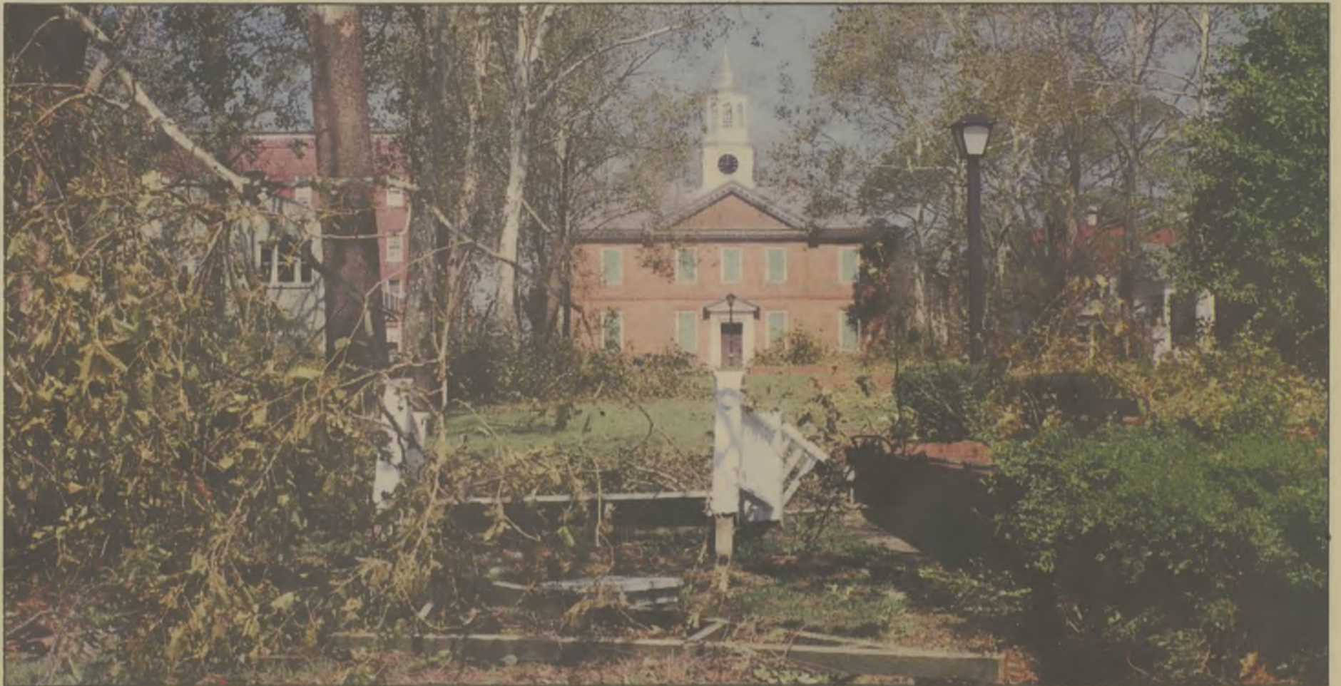
After the fury unleashed by Hurricane Isabel the historic Chowan County Courthouse still stands in stately elegance in stark contrast to the confusing jumble of broken tree limbs and twisted signage crumpled at the bottom of the Courthouse Green. (Staff photo by David Crawley)
