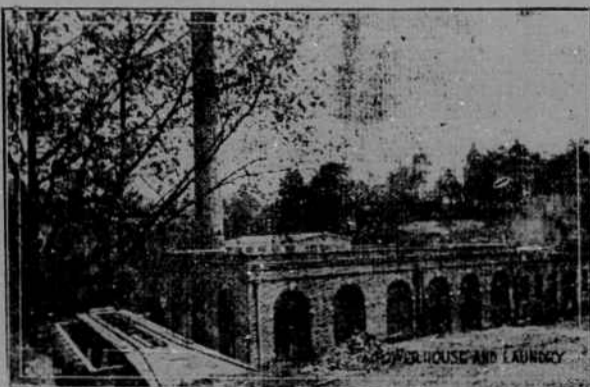
Powerhouse and Laundry With Madison Building Showing in Background
